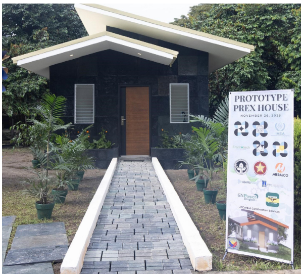
This residential house prototype is the first-of-its-kind model of a house built with radiation-processed plastic tiles, panels, and bricks. It's a product of a study that low-value plastic wastes can be turned into durable construction materials. (Photo by John Louver Patriarcha, DOSTv)
